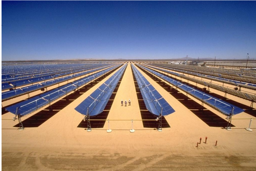
Figure 1.5: A broad view of parabolic trough solar collectors at Kramer Junction, California, USA [10]
