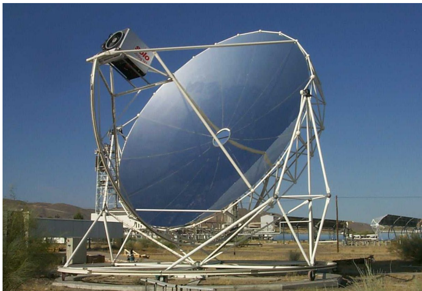
Figure 1.9: View of a parabolic dish solar system [27]
