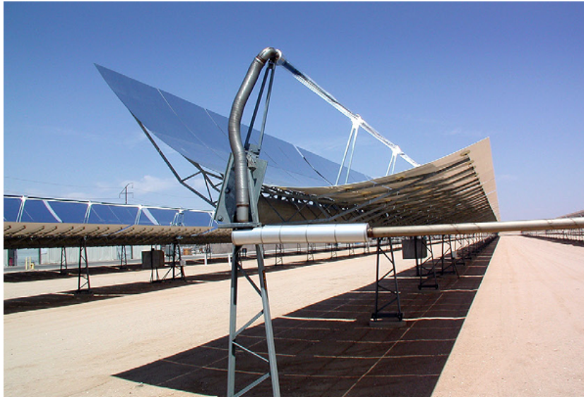
Figure 1.3: View of a parabolic trough collector [9]
