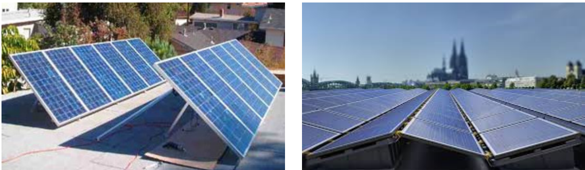
Figure 64: South and E-W frameworks
