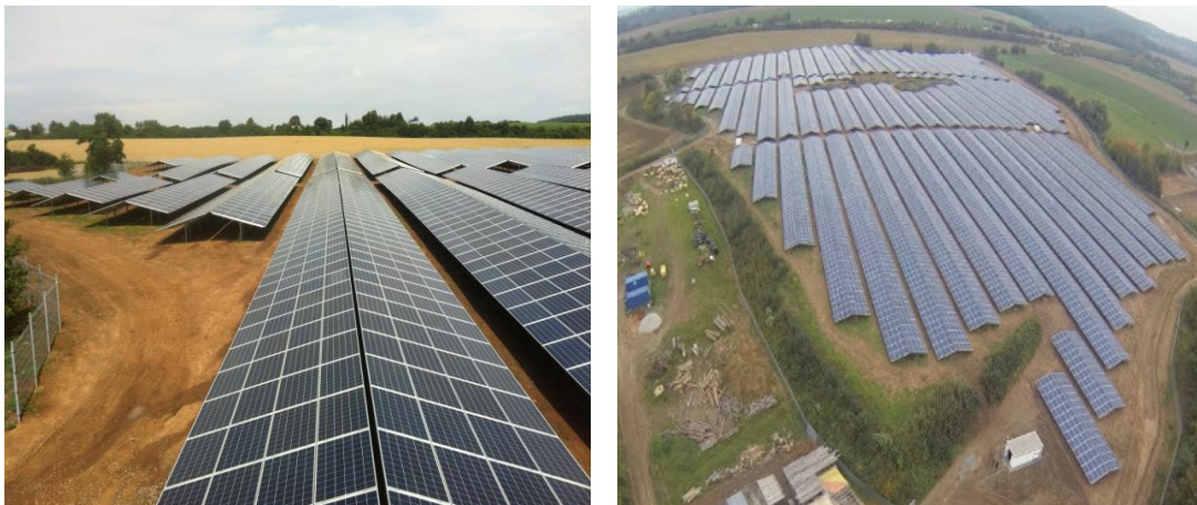
Figure 5: Photographs of the Hölzengraben project
