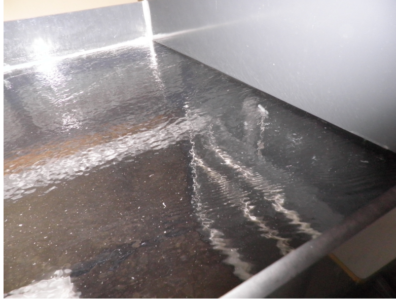
Pic. 15 Turbulences with the pumps working.
