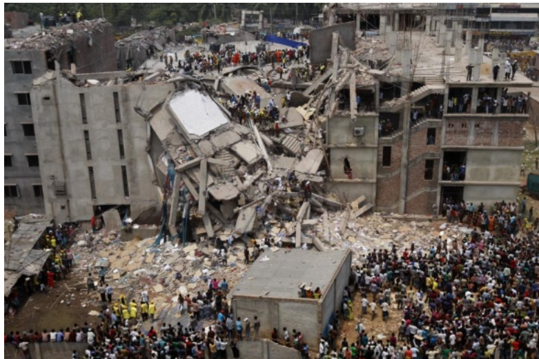
Figure 2 Rana Plaza building collapsed in 2013
