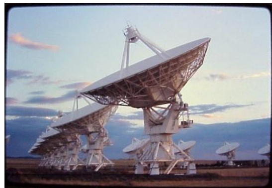
Figure 2.- VLA system picture. Each reflector includes at its focal plane the multiple feed configuration shown in figure 1.
