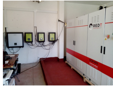
Figure 5: Vanadium Redox Battery demonstrator
