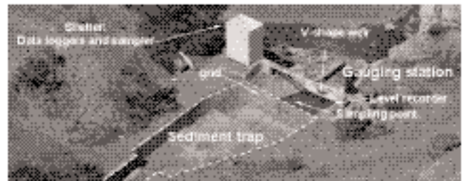
Fig. 2. Measurement device at the outlet of the basin.
