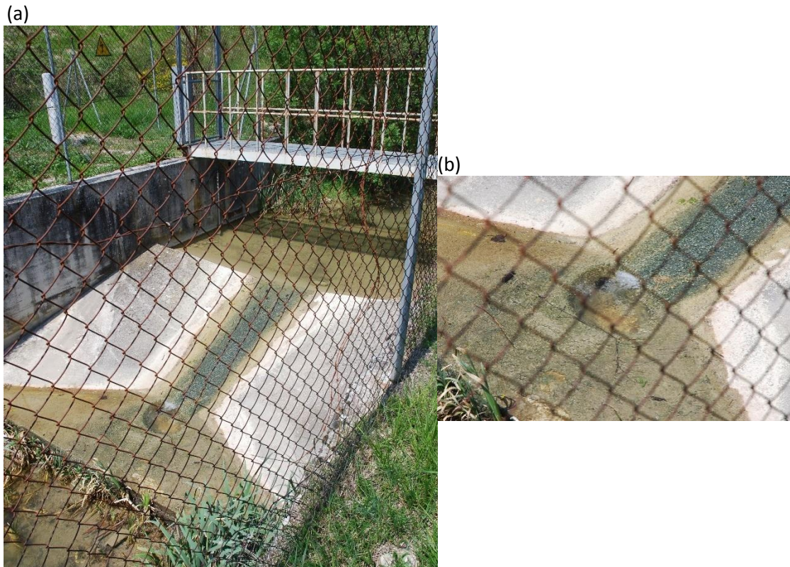
Figure 6. Pictures of the hydrological station from Latxaga watershed, exemplifying (a) the triangular profile flat-V weir and (b) the spherical hollow that takes the samples.
