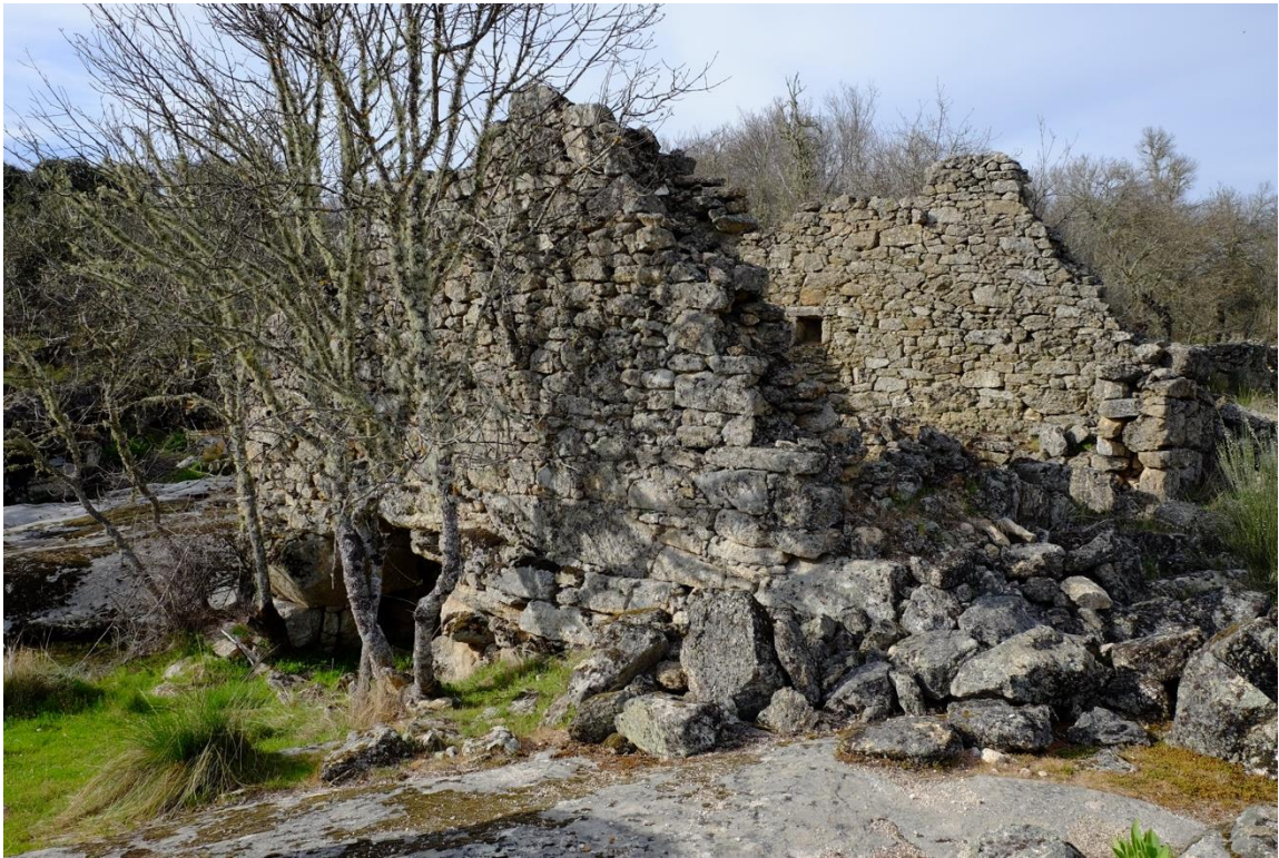
Fig. 5a. Ruined stone watermill in southwest Ifanes municipality
