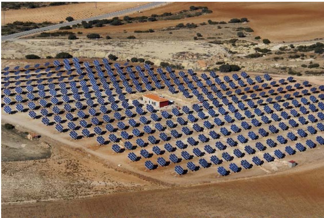
Figure 1: Example of installation. Photography by solar garden located in Bonete (Spain). [17]
