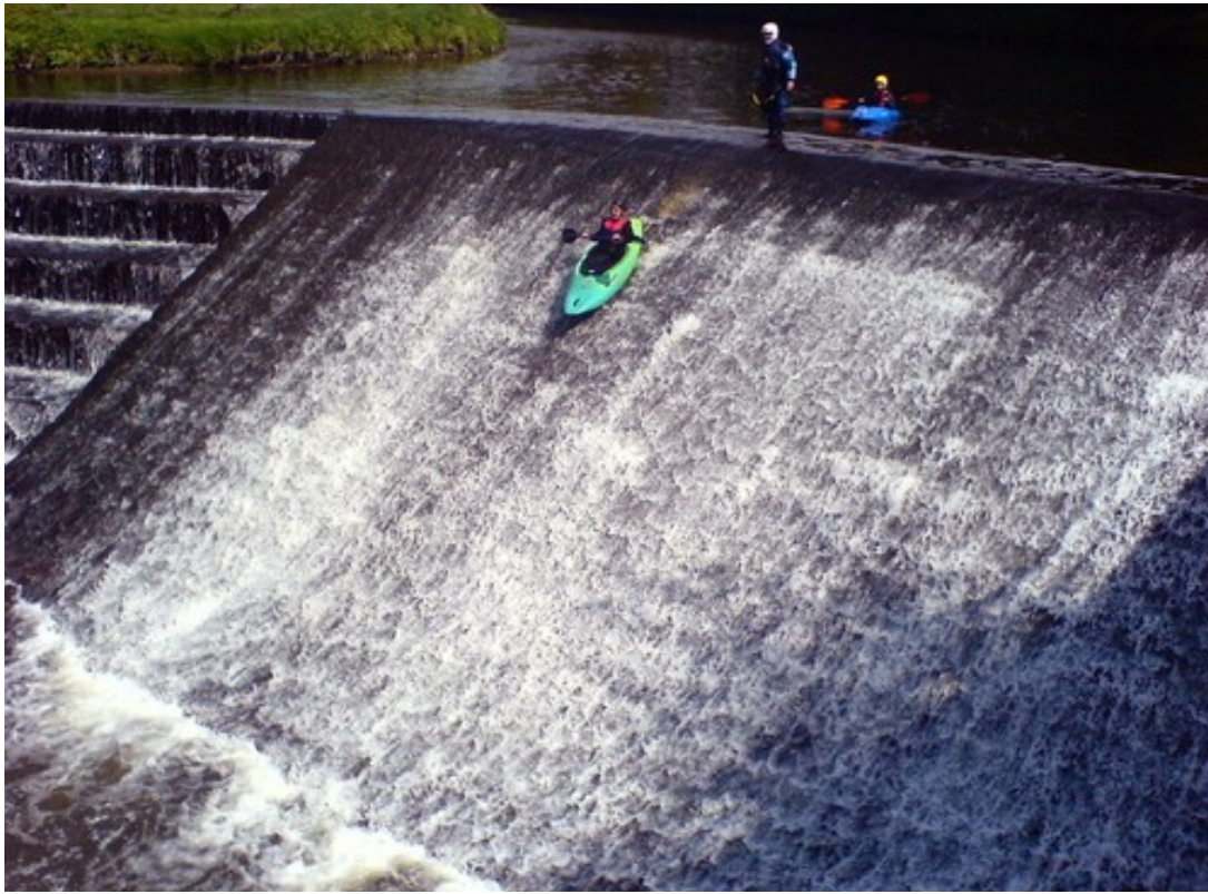
Figure 6, Burrs weir photo (panoramio, 2012)
