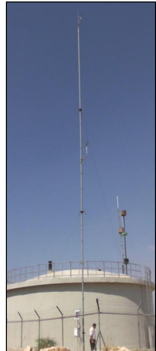
FIGURE 4: WEATHER STATION IN TUBAS
