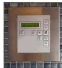
Panel de control.
