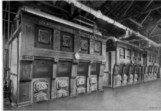
Image 2 - Stirling boilers (Philadelphia and Columbia).
