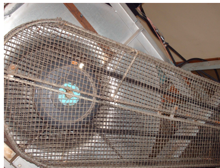
Figure 5: The belt and the two pulleys
