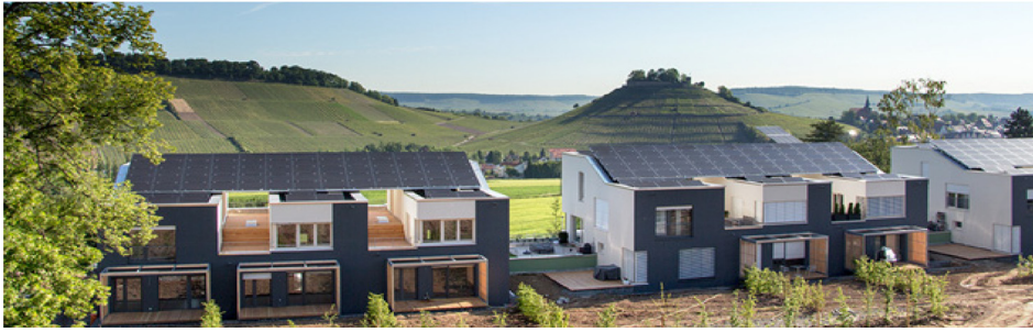
FIG. 1. Picture of the residential neighborhood in Weinsberg, Germany. The combination of PV modules, a CHP engine, and energy storage systems allows a high level of self-sufficiency in the energy consumption of the neighborhood. Reproduced with permission from DSG Holding GmbH & Co. KG.
