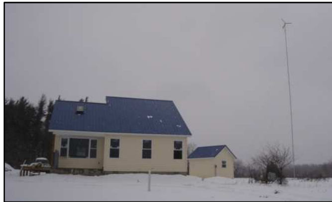
Figure 13. Installation in an insulated building
