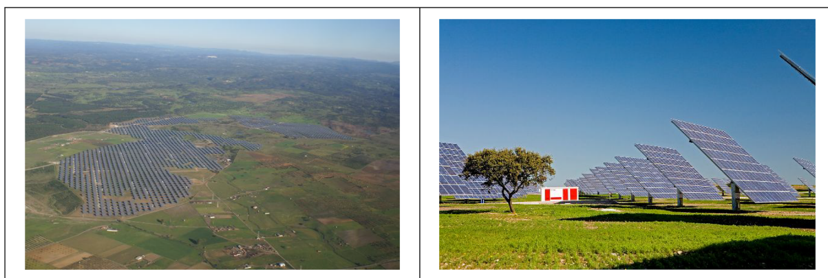
FIGURE 2 PV plant P13, with 46 MWp, was installed in 2008. It is composed by 134 m 2 trackers. Each group of 36 trackers is connected to a 500- kW power station, having one only selling contract for the whole plant
