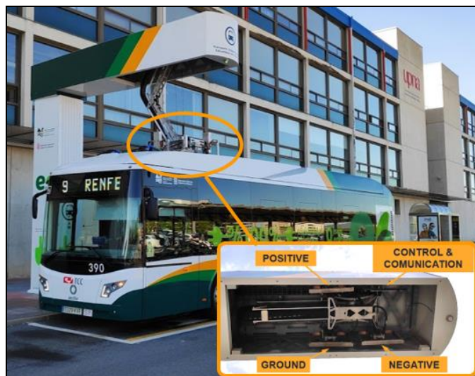
Fig. 2. Bus charging station at Public University of Navarra Campus.
