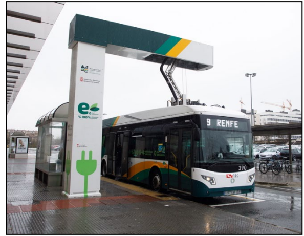
Fig. 1. Bus fast-charging point at UPNA.
