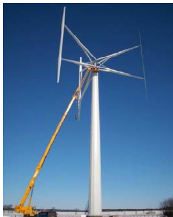
Figure 4.7: VAWT in Falkenberg, Sweden.
