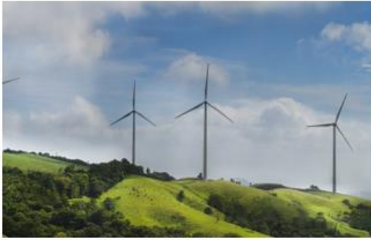
Project: ALISIOS Wind Farm Scope: Civil supervision during construction Location: Costa Rica
