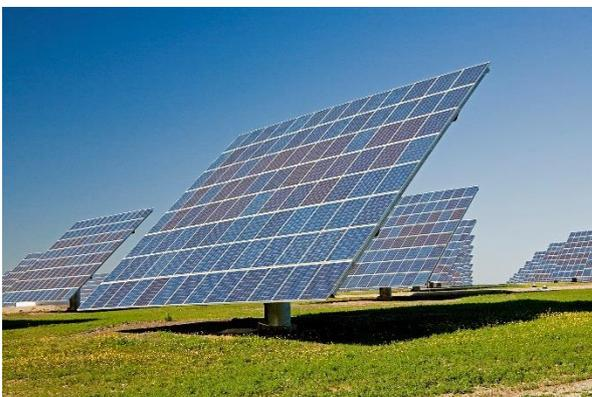
Fig. 2.3 Seguidor Azimutal.
