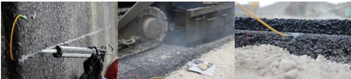
Fig. 3. Pictures of the sensing fibers installation, the second layer paving procedure and resulting interface.
