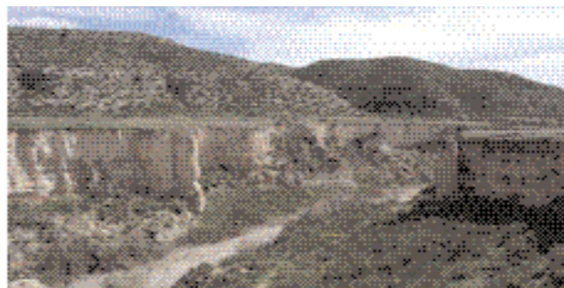
Fig. 1. Gully in the Barranco de Alfocea .
