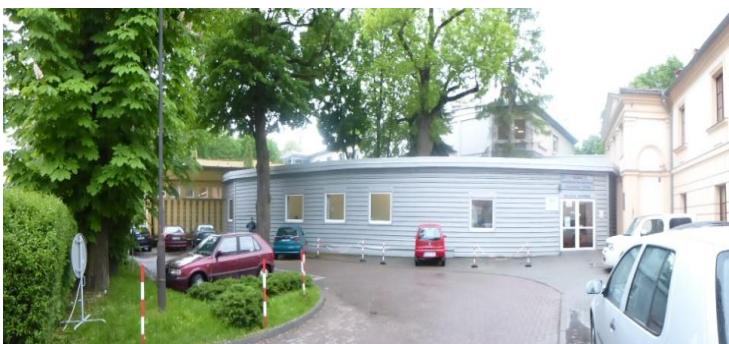
Figure 2: Hospital of Krzeszowice temporary part (Tornos U. and Villegas R.)
