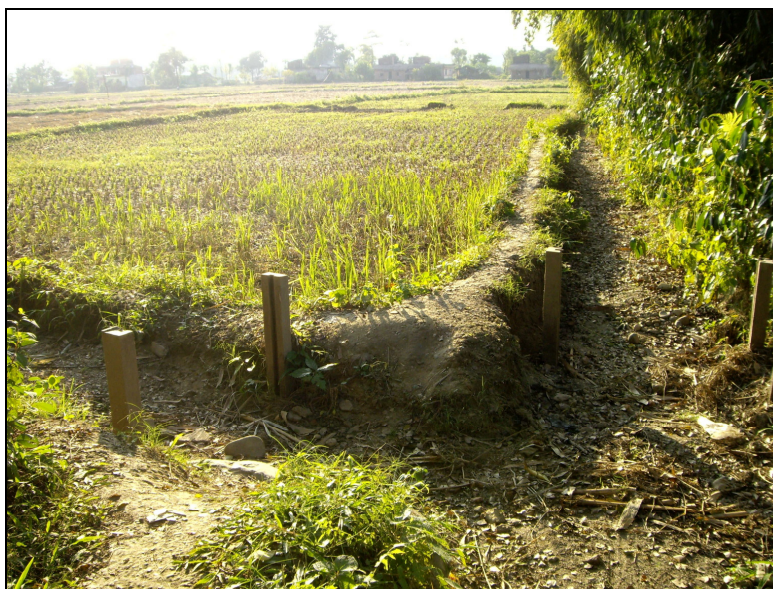
Image 3: Common Branch and Sub-Branch canal features with earthen lining and embankment.
