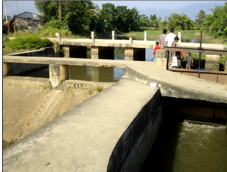
Image 1 PIS Headworks, note PIS intake's sluice gate (right).
