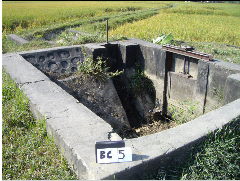
Image 5: BC5 sub-branch diversion structure
