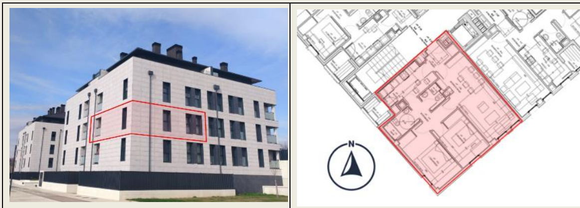
Figure 82. Picture of the south-east, south-west facades of the case study building with 21 dwellings.
