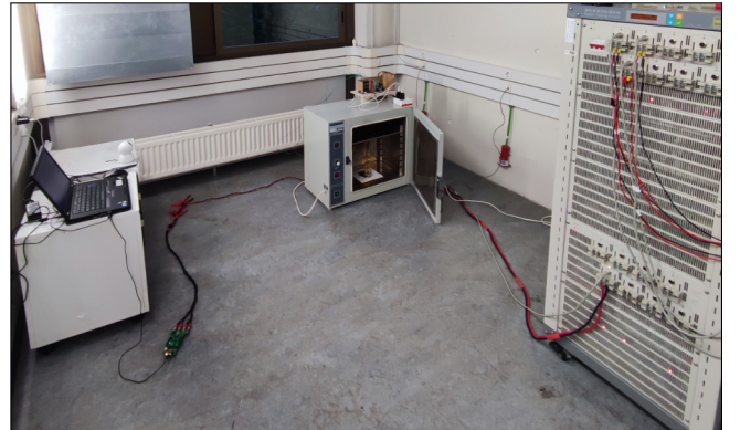
Fig. 4: Experimental test bench in the Laboratory for Energy Storage and Microgrids of the Public University of Navarre.
